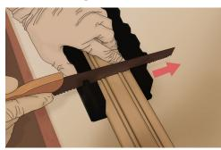
Use tape-measure or roulette to measure surface a molding will be applied to. Calculate a required number of profiles precisely. Cut off a profile excess to fit your dimensions. Use miter box to make accurate angled cuts.
