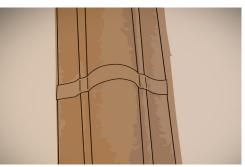
When it is perfectly dry, fill the joints with the flexible Molding Creator putty. Use fine-grained type for filling internal profiles and coarse-grained for outside ones. Put the mass with a putty knife and fill joints carefully. Use it at ambient temperature of 50 °F to 88 °F. Wait until it is totally dry.
